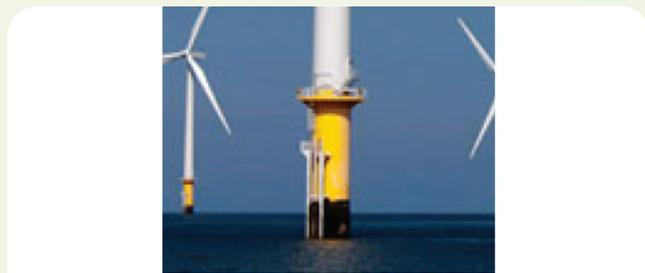
Figure 11. A typical monopile foundation
