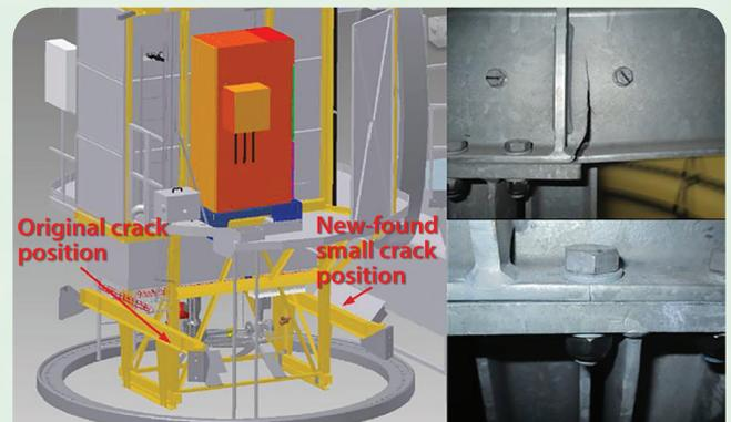
Figure 5. Internal space frame cracking
