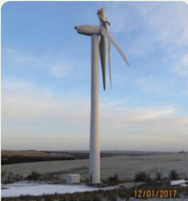
Figure 6. Example of a recent blade failure
