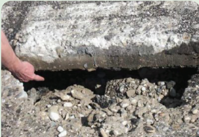
Figure 26. Example of an air pocket that can be detected using muons
