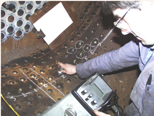
Figure 12. Ultrasonic testing of stays after surface preparation
