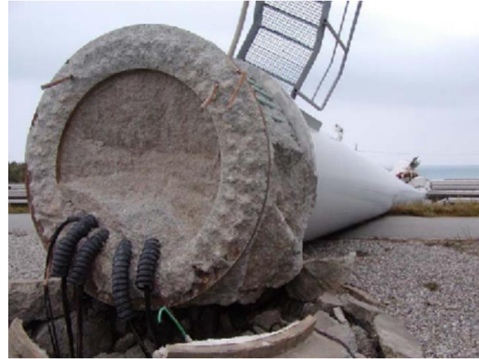
Damage caused by typhoon Maemi in 2003 (Ishihara et al, 2005)
