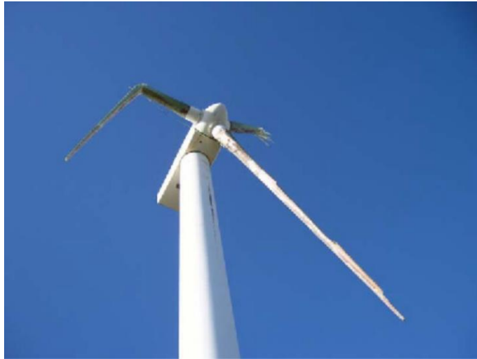
Damage caused by typhoon Maemi in 2003 (Ishihara et al, 2005)
